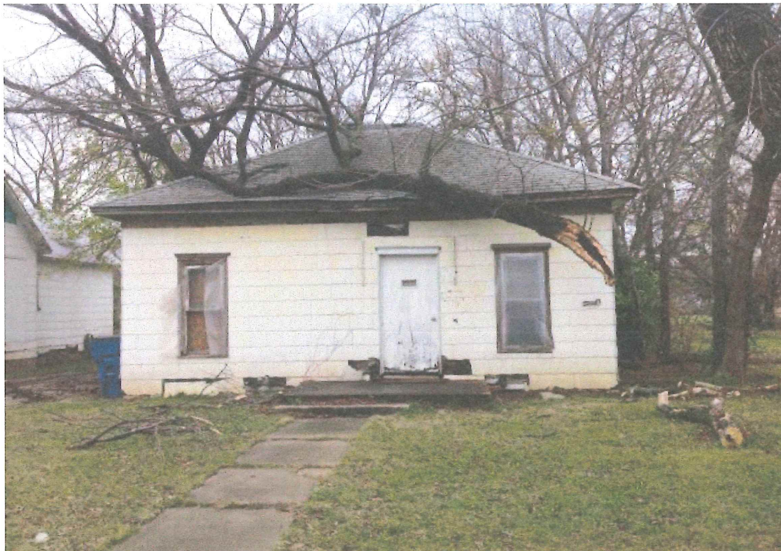
@ 910 square feet single level dwelling.
