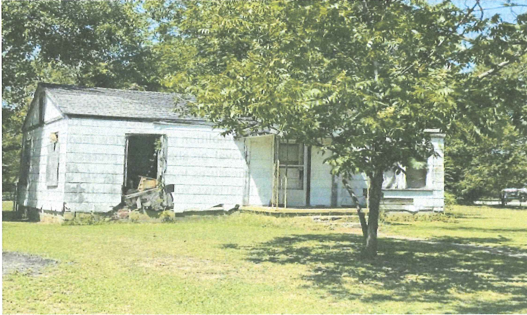
@ 640 square feet single level dwelling.
