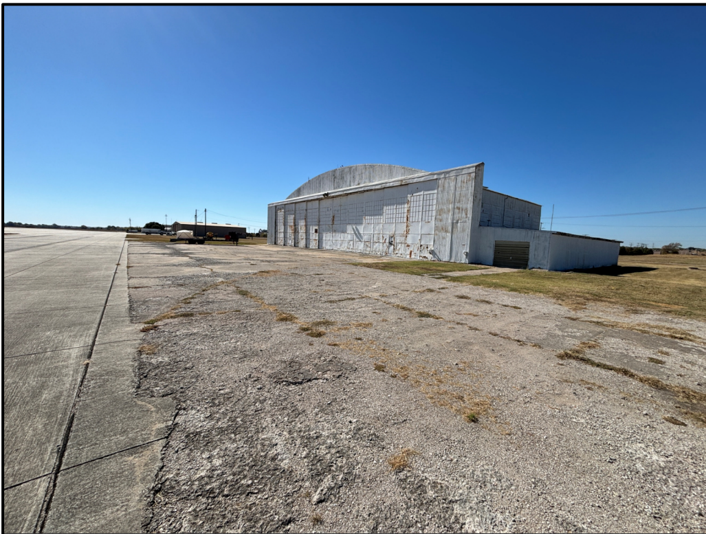
Existing Condition of Hangar Approach
