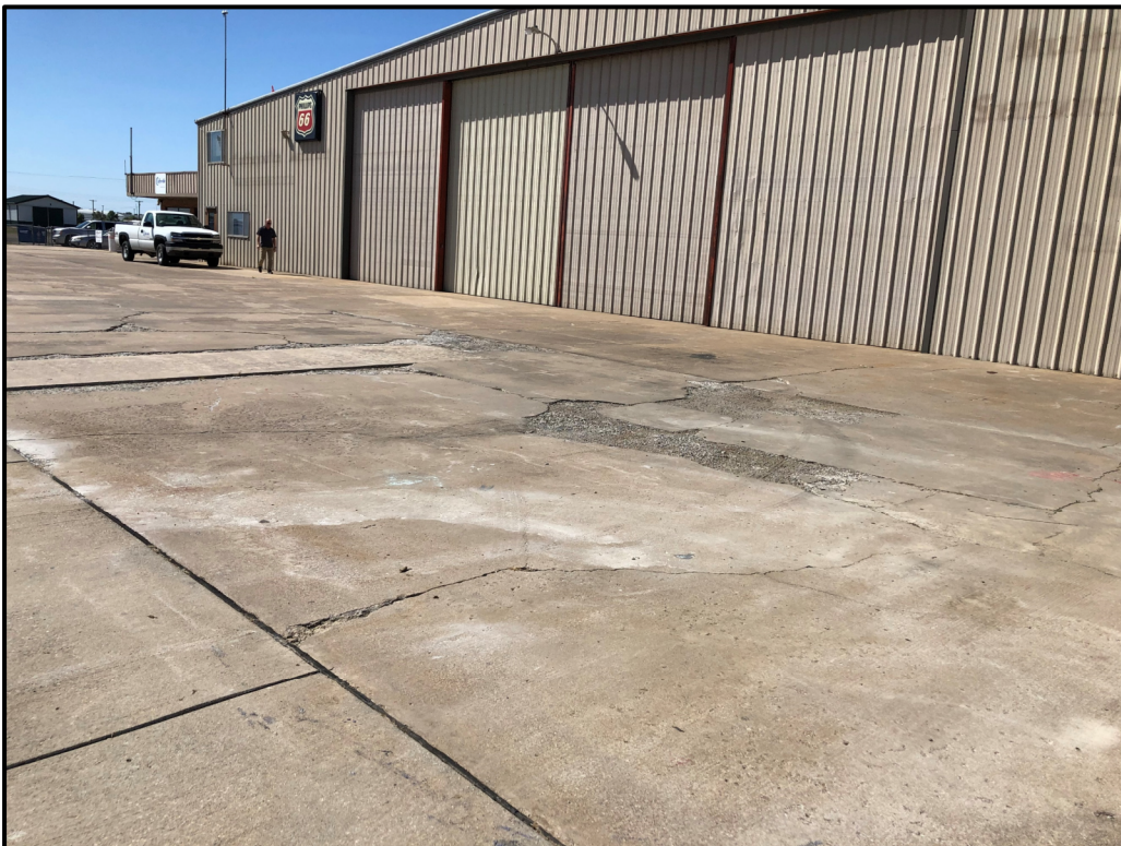
Existing Condition of Hangar Approach
