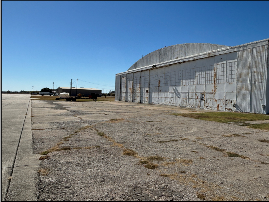
Existing Condition of Hangar Approach
