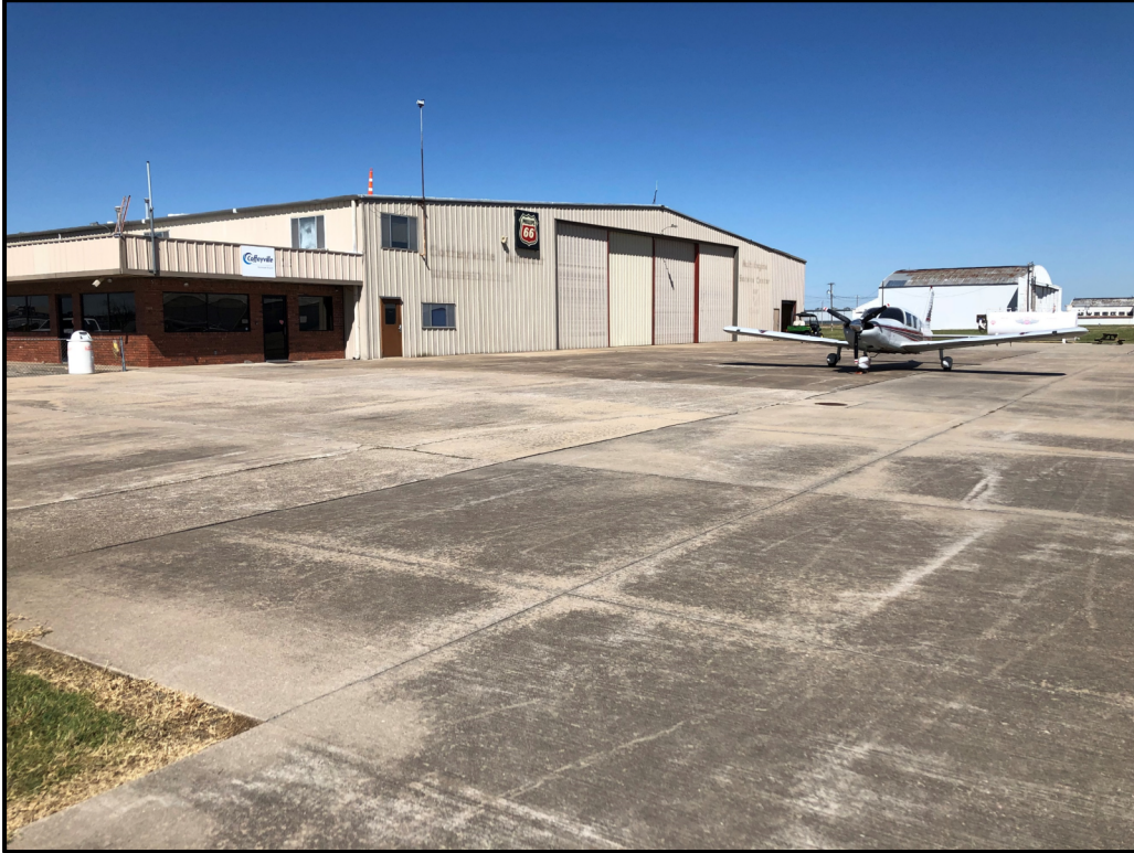
Existing Condition of Hangar Approach
