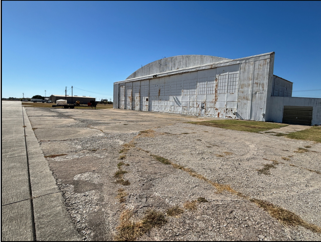
Existing Condition of Hangar Approach
