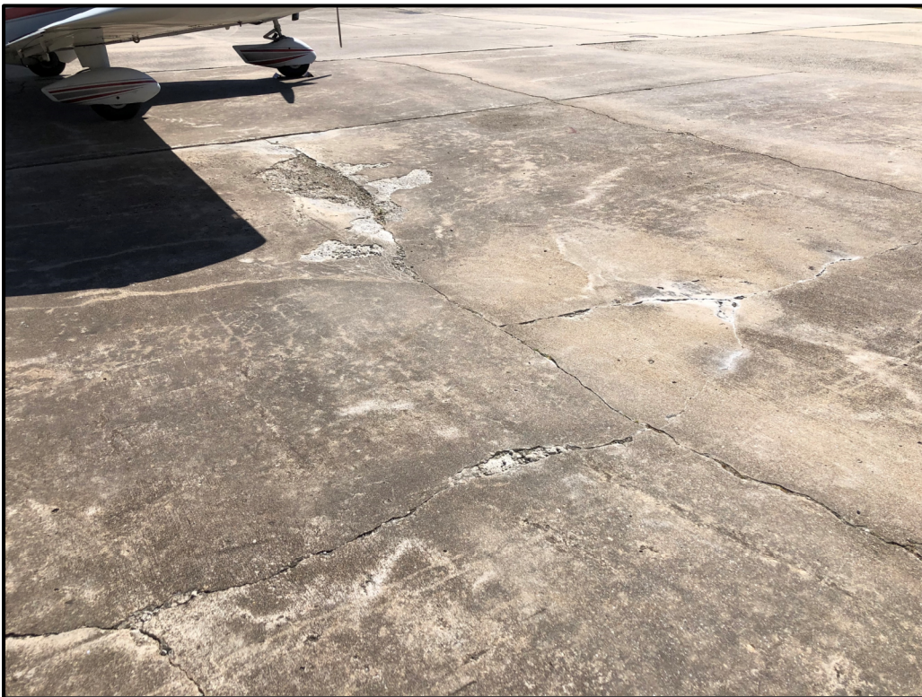
Existing Condition of Hangar Approach
