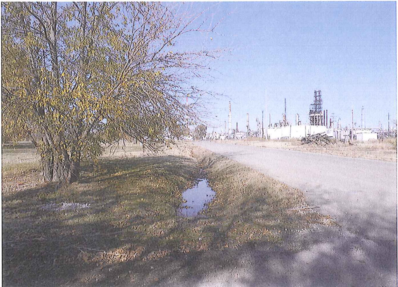
View of Site from New Street, looking North at Sparks Street
