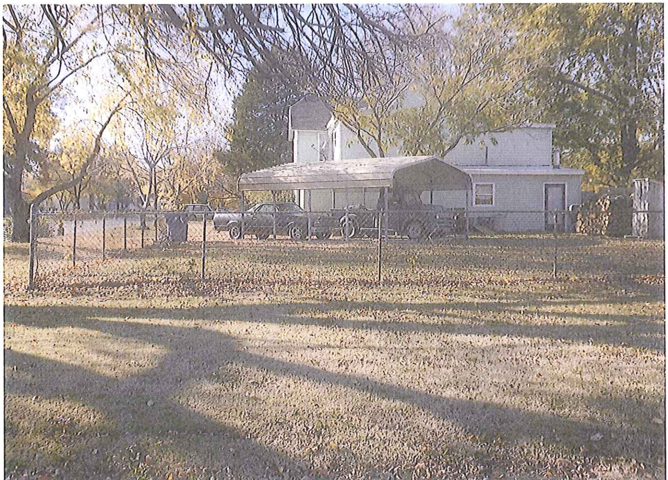
View from Site looking West from Union Street at New Street
