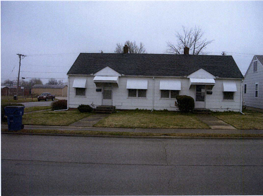
View of Site From North
