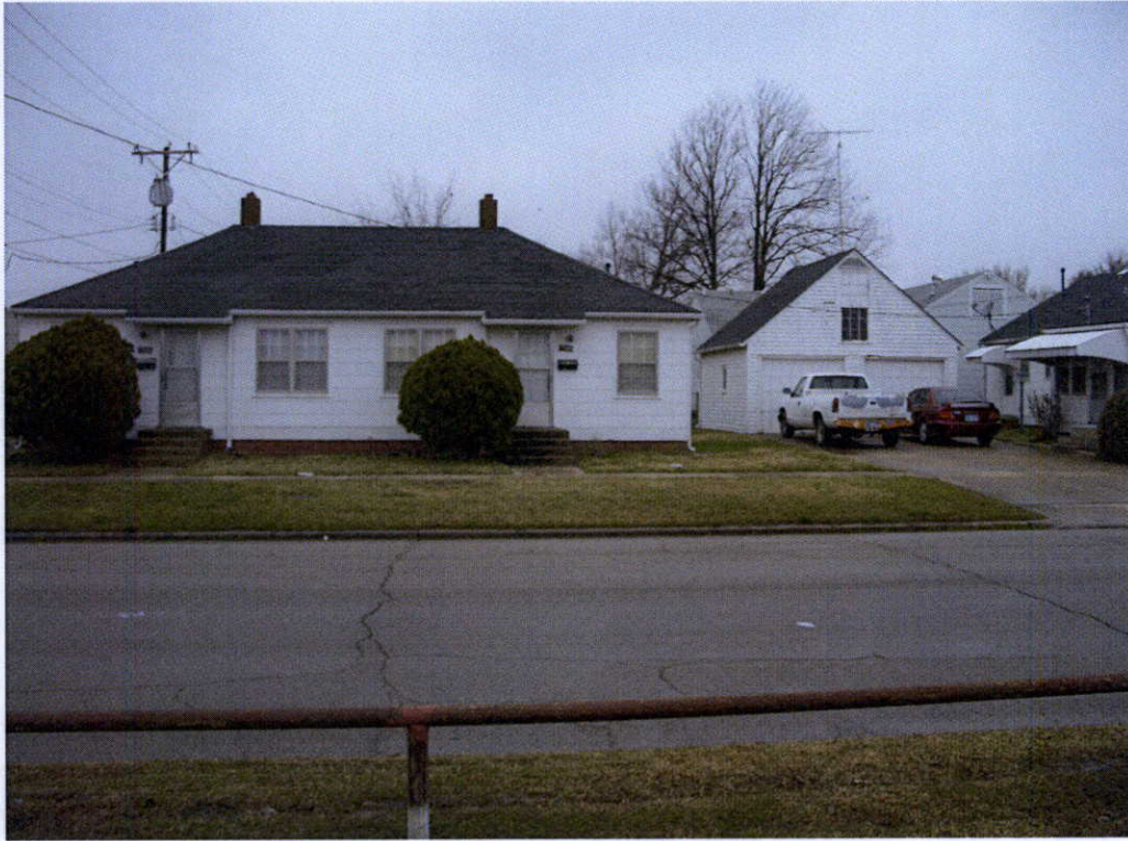
View of Site From East
