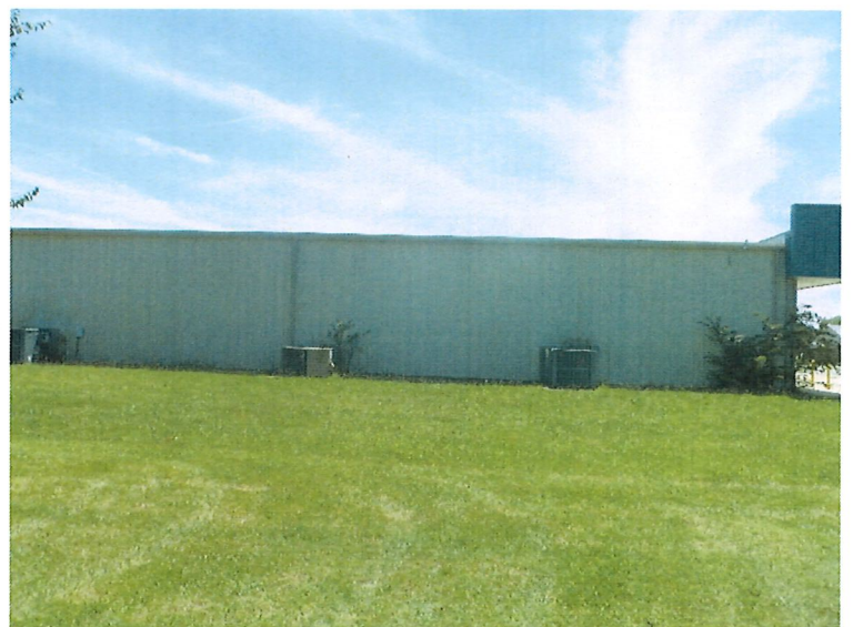
Looking at property from the North
