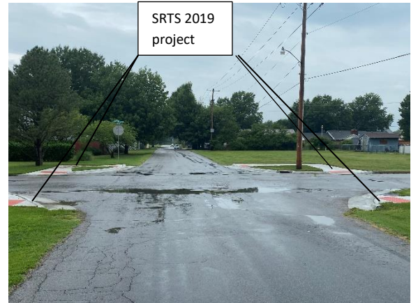
10. West on Northfield @ Parkview
