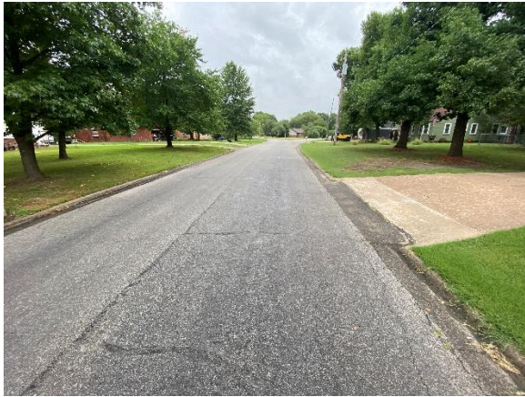
3. North on Highland near Parkway
