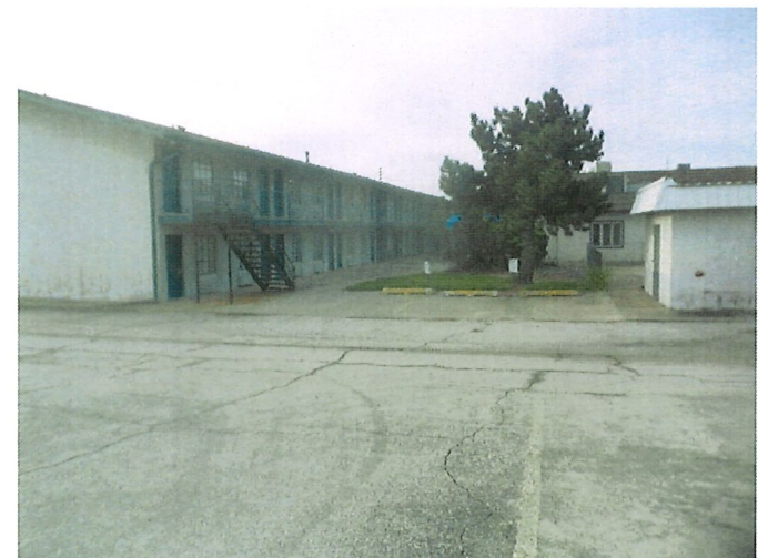
Looking at property from North #2
