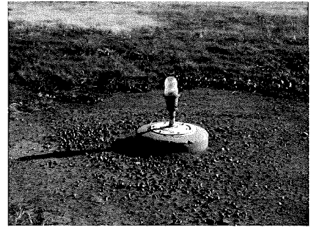
Runway Light Prior to Installation of Protection Ring
