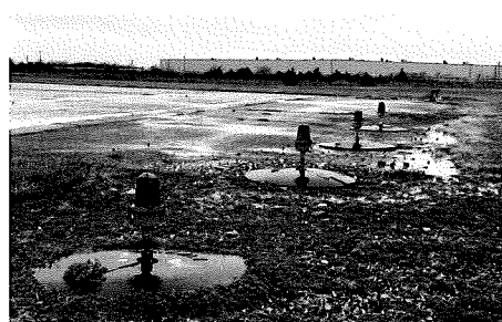
Existing Runway 17-35 Threshold Lights
