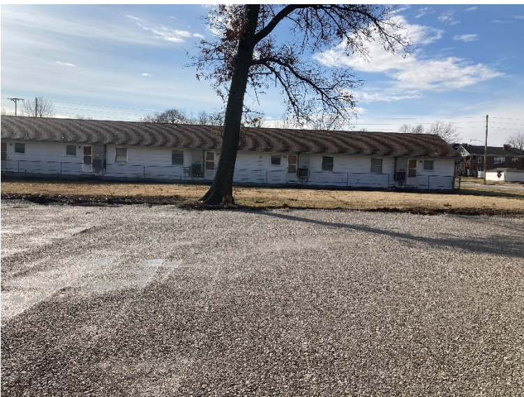
Looking South from the property
