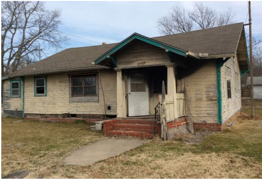
Non-friable Window Glazing – located on exterior
